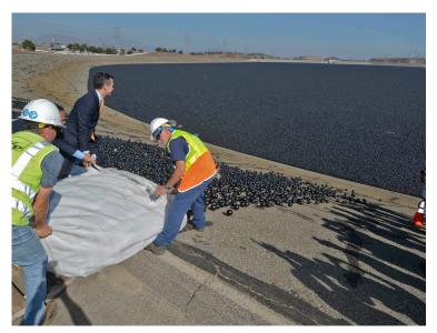
away by wind gusts, as the reservoir is located in a high gust area. Shade balls in place at other LA reservoirs - Elysian, Ivanhoe and Upper Stone Canyon - are hollow and not filled with water.
