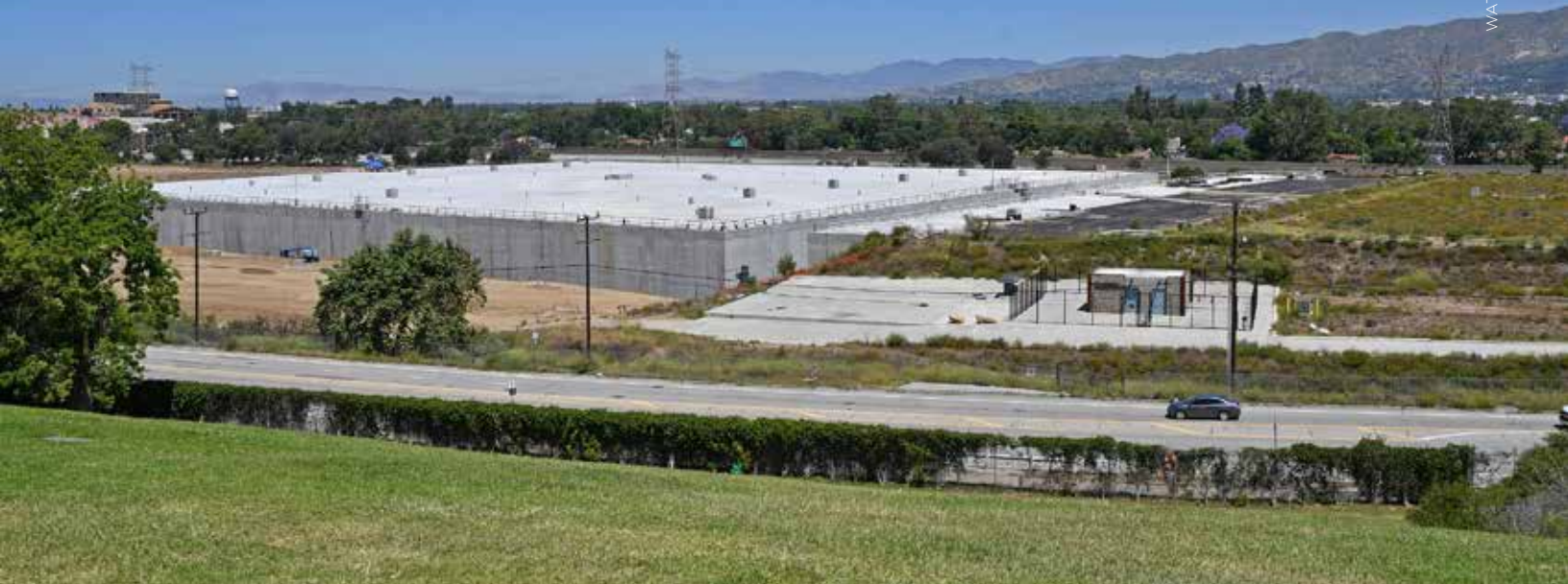
Headworks Reservoir Complex
