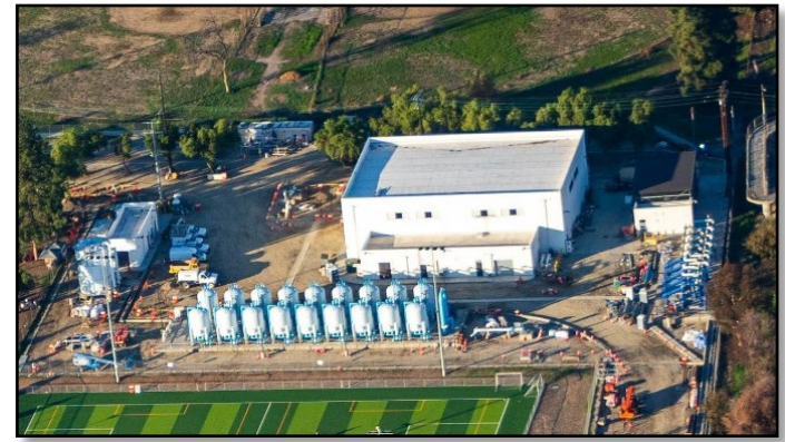
North Hollywood West (NHW) Treatment Facility
