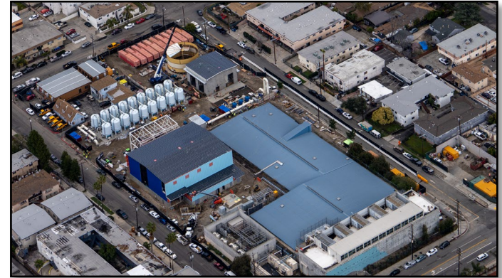
North Hollywood Central (NHC) Treatment Facility
